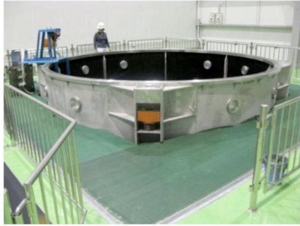
Stainless Steel Vessel (SSV) in assembly pit
